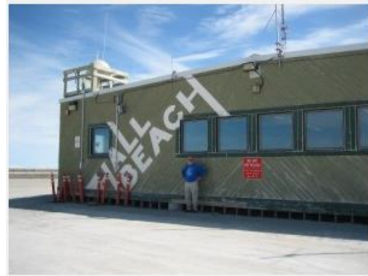
In 1960, the 'terminal building' was an USAF blue school bus.
