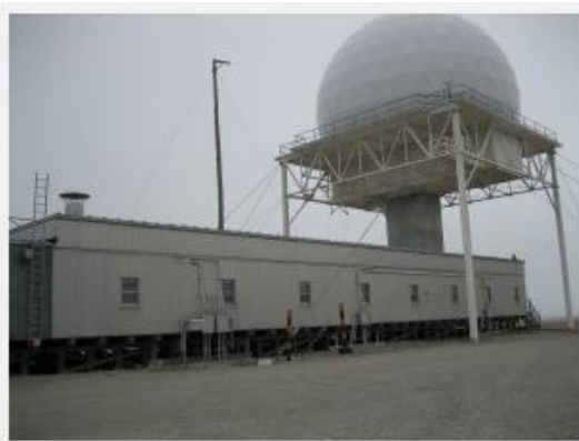
The Electronics modules were where I spent much of my working life while on the Line.
