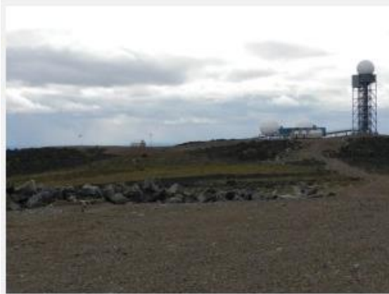
CAM-4 is no more and was replaced by CAM-4A as seen from the old CAM-4 site.
