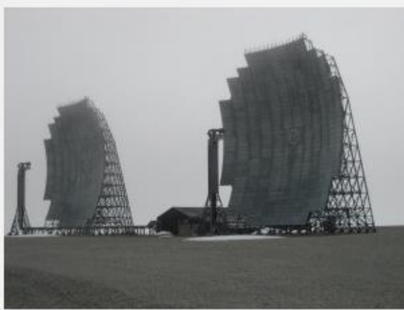
90 foot Tropo Antennas. Note the size of the equipment building at the base.
